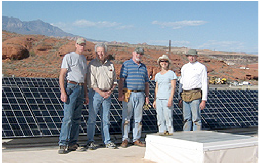
(Left to right) City of St. George employees Gerald Whipple and Orrin Farnsworth join installers Jeff Pomeroy, Sara Baldwin and Brian Smith to celebrate the completion of the 5-kW solar array the city installed on its Water and Energy Administration building. (Photo by Ken Gardner)
