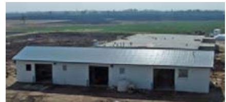
Midwest Dairy Institute's covered digester, above, collects and processes waste from 1,400 cattle into bedding, fertilizer and biogas to power a fuel cell, below. (Photo by Midwest Dairy Institute)
