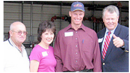
osie and Danny Kluthe (center) were joined by Nebraska state senators Arnie Stuthman (left) and Matt Connealy to cut the ribbon on the Kluthes' digester gas-powered generator, the first in the state. (Photo by Cuming County Public Power District)
