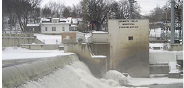
The city-owned, 1.2-MW hydroelectric dam on the Minnesota River helps Granite Falls Municipal Utilities to provide low-cost electricity to residents. (Photo by Granite Falls Municipal Utilities)
