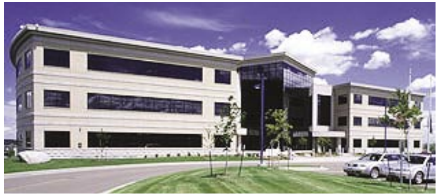
Large windows on the north face of Century Center wed aesthetics and efficiency by bringing natural light into the office building. (Photo courtesy of Steve Silverman, Grand Forks, N.D.)
