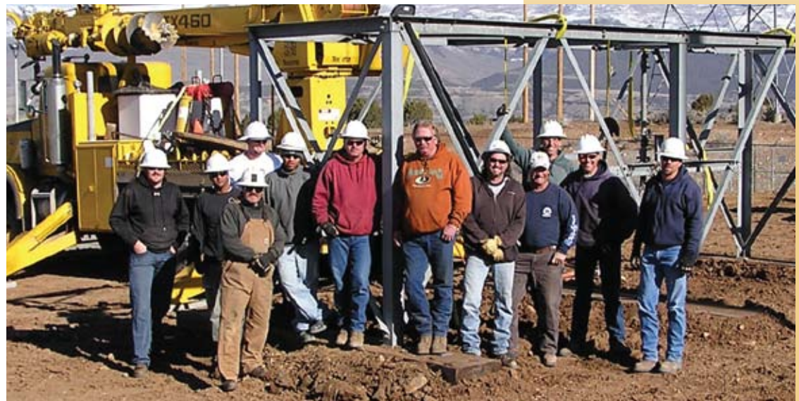
Line crews from Montrose, Cheyenne and Phoenix combined efforts to install a shoo-fly for Tri-State Generation and Transmission.
