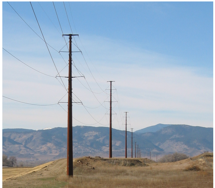
A COR-TEN® finished “Horizontal Vee” pole type is shorter and narrower than the original pole design.
