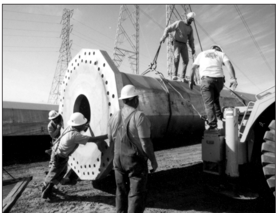
A construction crew maneuvers the base section of a steel pole.
