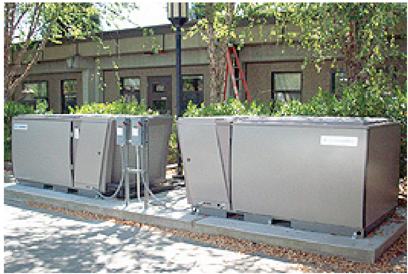
The combination of a 1.2-MW solar system and six Ice Bear cooling systems reduces Napa Valley Community College's peak power consumption by more than 1.5 MW. (Photo by Ice Energy LLC)
