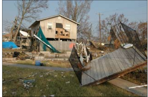
Biloxi, Mississippi, September 3, 2005 -- Damage and destruction to houses in Biloxi, Mississippi, after Hurricane Katrina (Mark Wolfe/FEMA photo)
