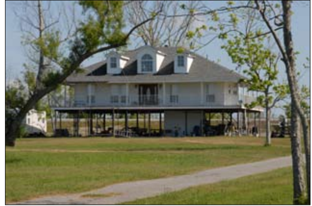
Port Sulphur, Louisiana, April 14, 2006 -- This is a "post" mitigated home that was raised up above the flood plain. The FEMA Mitigation program is designed to minimize loss through raising homes above the flood plain in flood-prone areas. (Marvin Nauman/FEMA photo)
