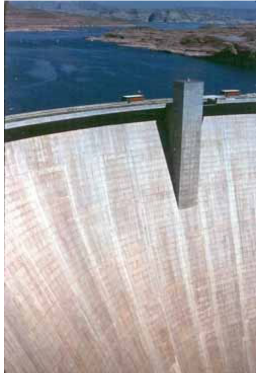
Figure 13. The U.S. has over 5,500 large dams
