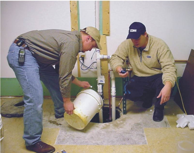
Figure 8-6. Testing pumping rate to support monitoring of a disconnected footing drain.
