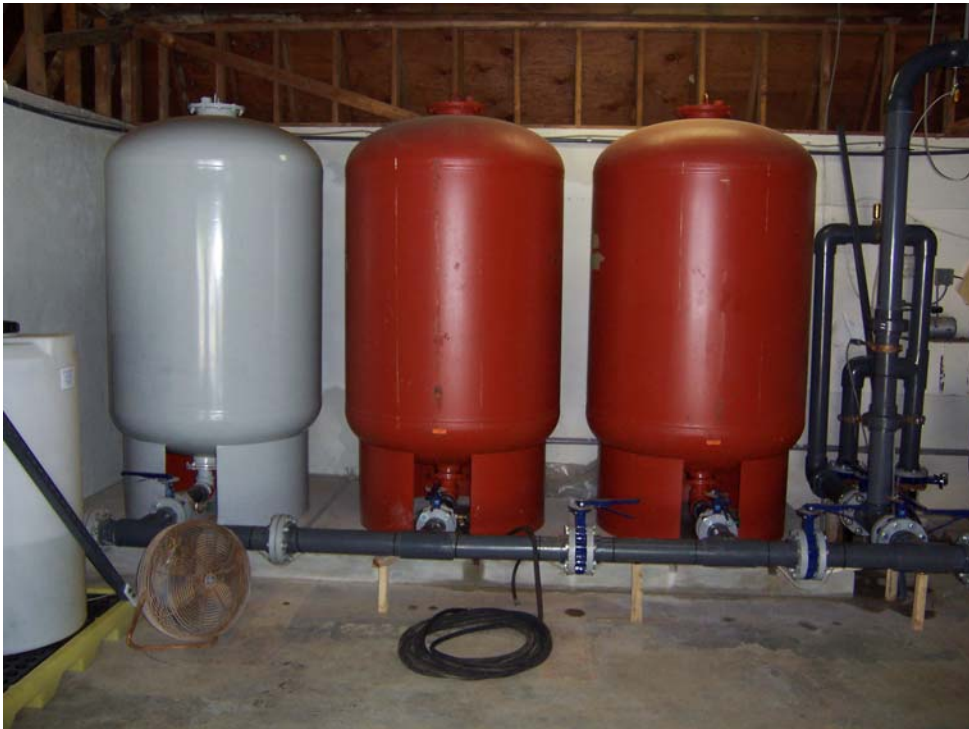
Figure 4-8. Hydropneumatic Tanks
