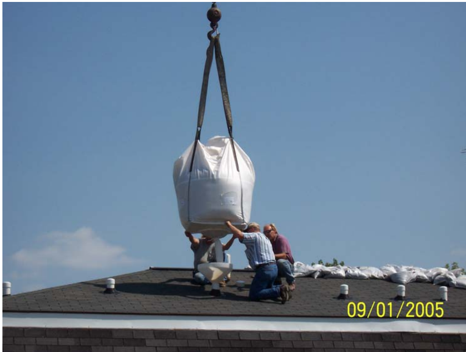
Figure 4-11. AD-33 Media Loading
