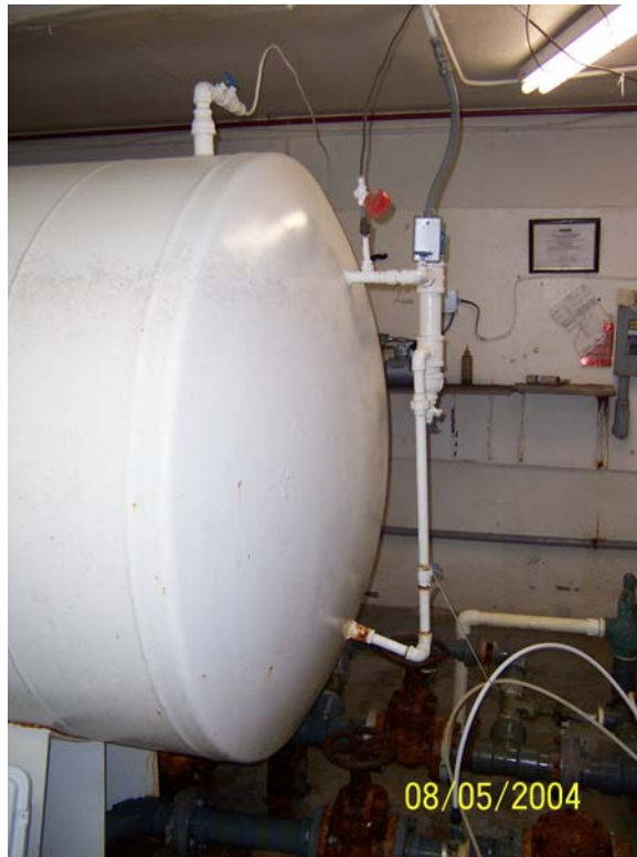
Figure 4-3. Preexisting Storage Tank
