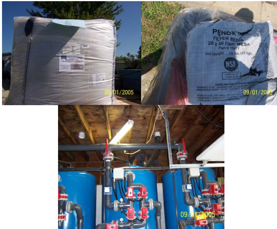
Figure 4-12. AD-33 Media Supersack, AD-26 Media Bags and Loading of Underbedding
