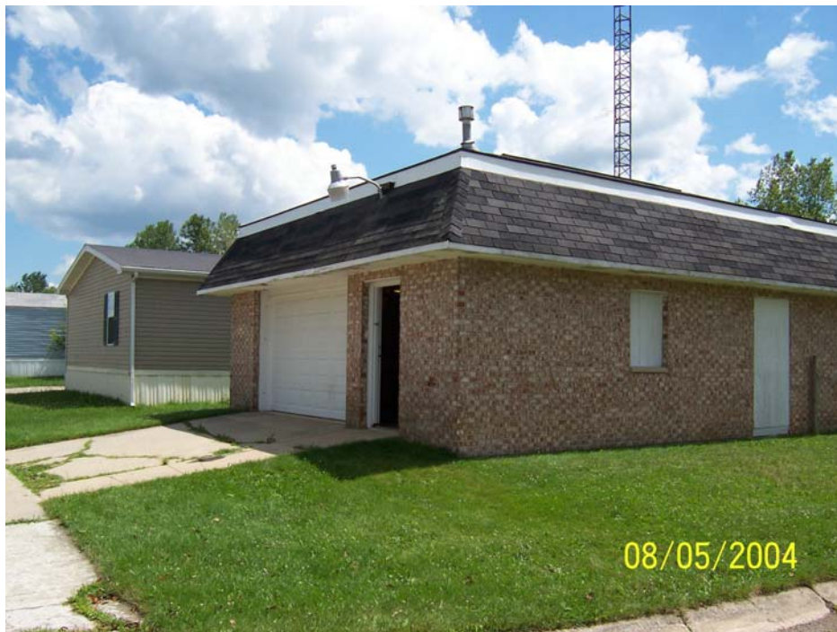
Figure 4-1. Preexisting Treatment Building at Chateau Estates Mobile Home Park
