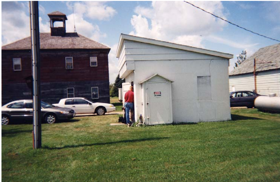
Figure 4-1. Pre-Existing Pump House at Climax, MN, Site
