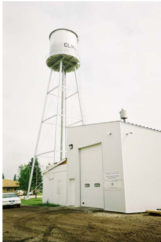
Figure 4-7. New Building Constructed Adjacent to the Pre-Existing Pump House and Water Tower
