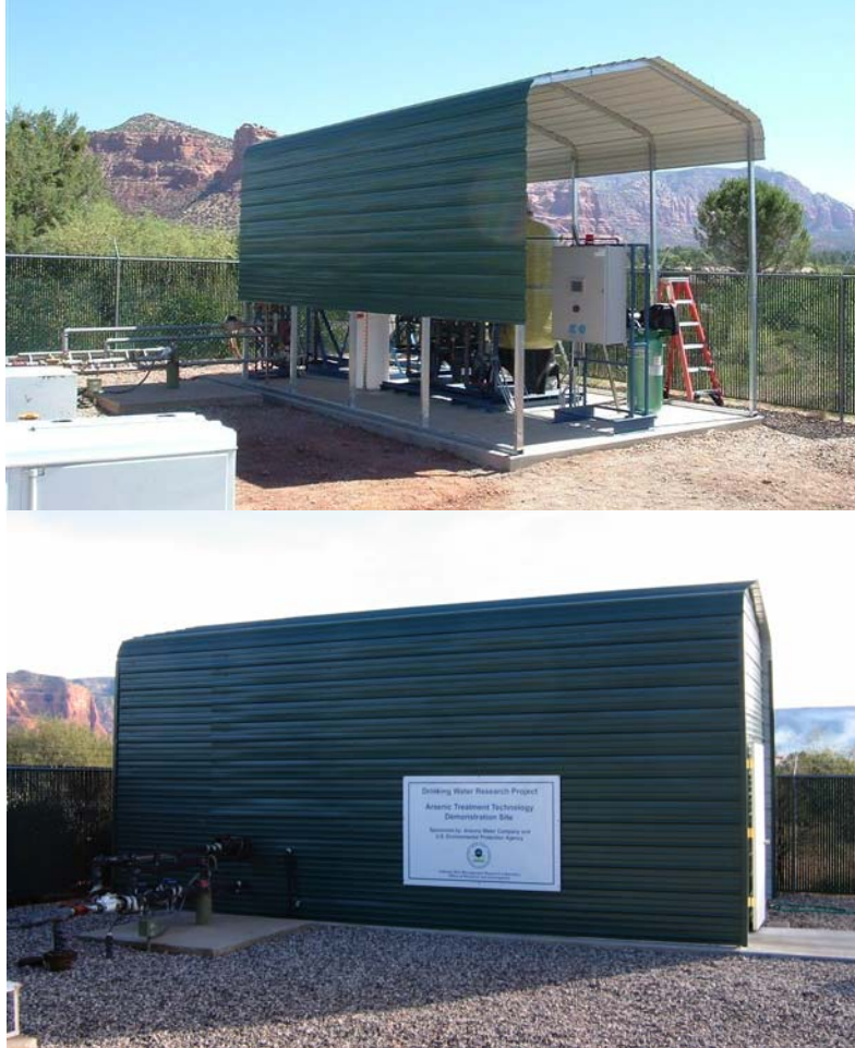
Figure 4-7. Sun Shed Structure (Top) and Completed Enclosure (Bottom)
