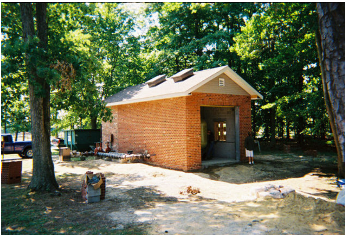
Figure 4-5. New Treatment Building Addition with Two Access Hatches in the Roof
