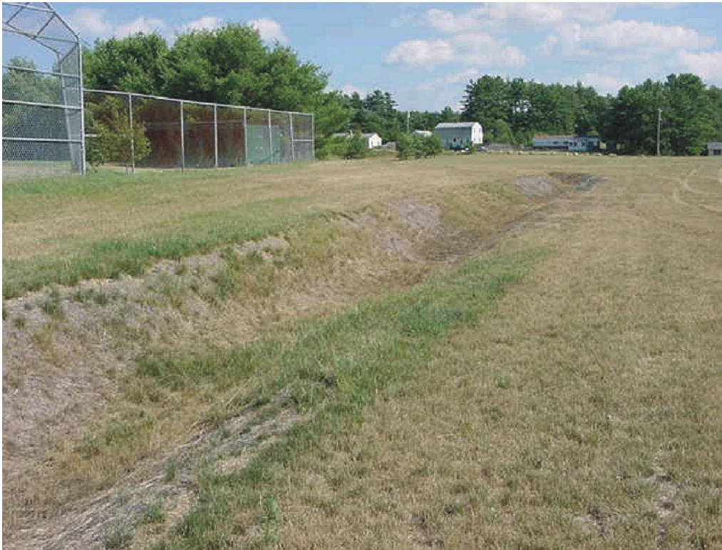
Drainage Culvert on the Site
