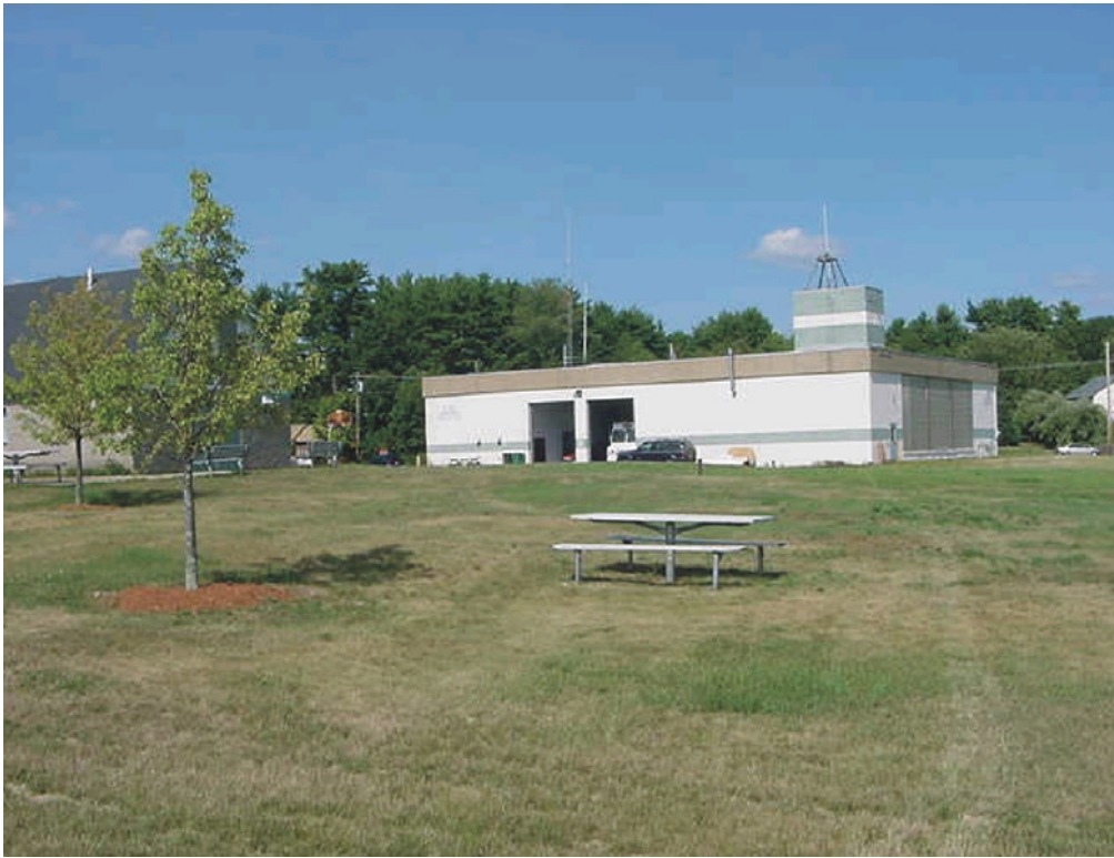
Fire Rescue Building on the East Side of the Site
