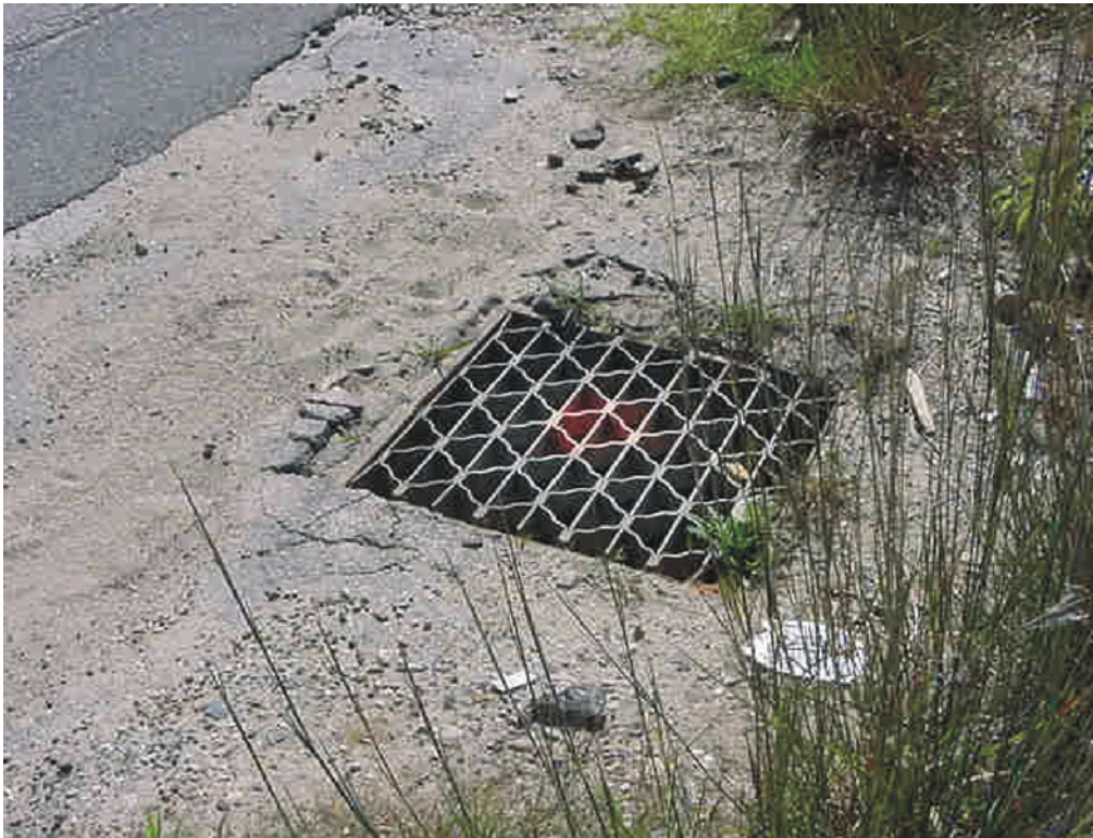
Storm Water Drain on the Somersworth Site
