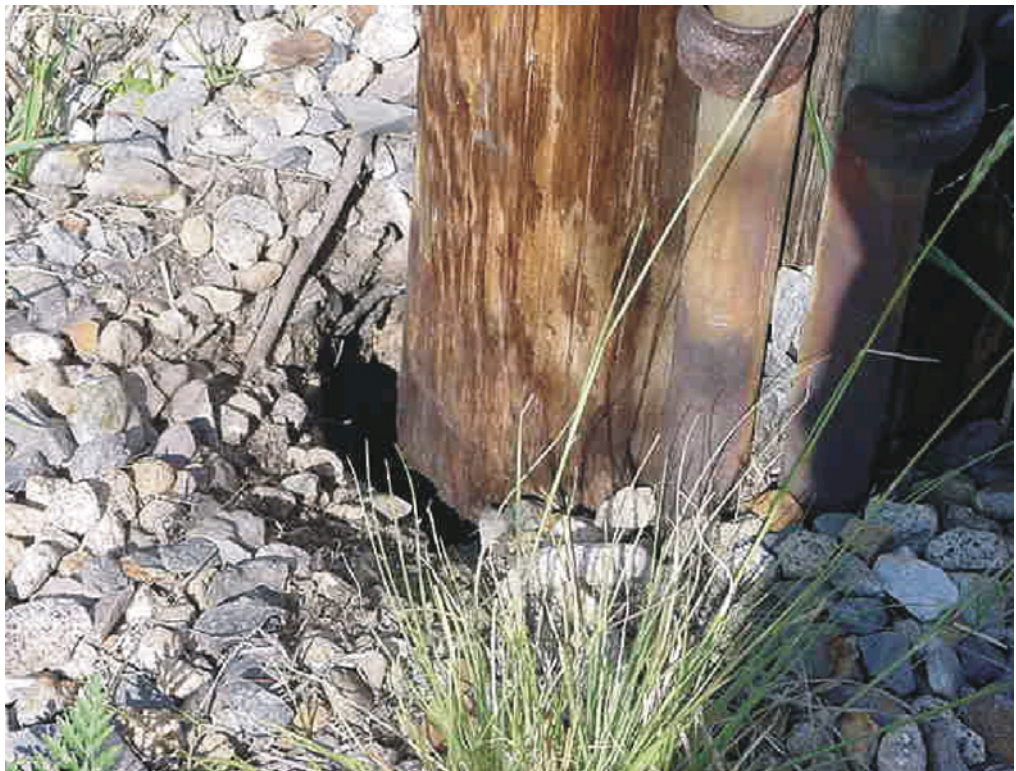
Base of the Tennis Court Light Poles
