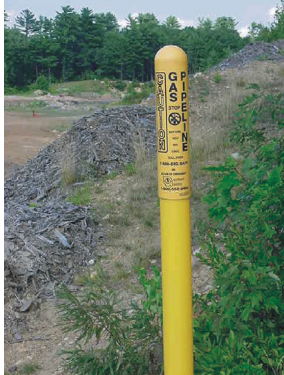
Gas Line Marker on the Somersworth Site
