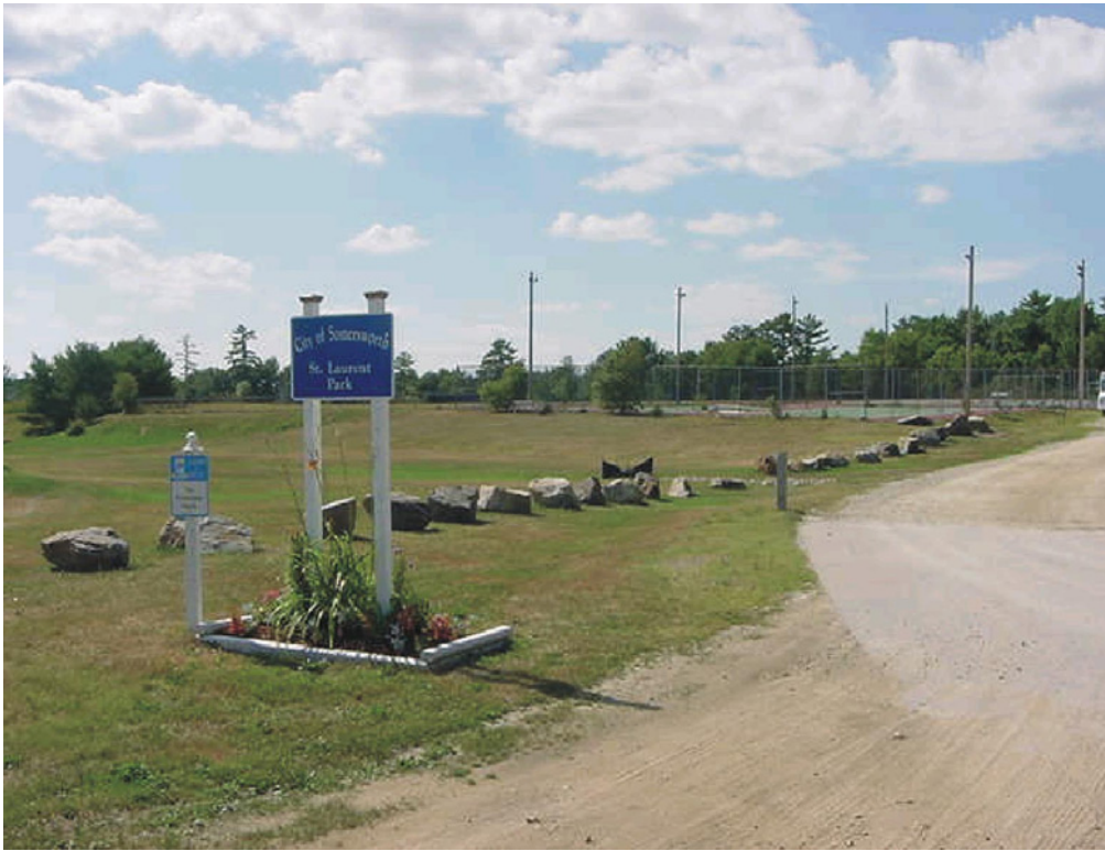
Somersworth Superfund Landfill Site
