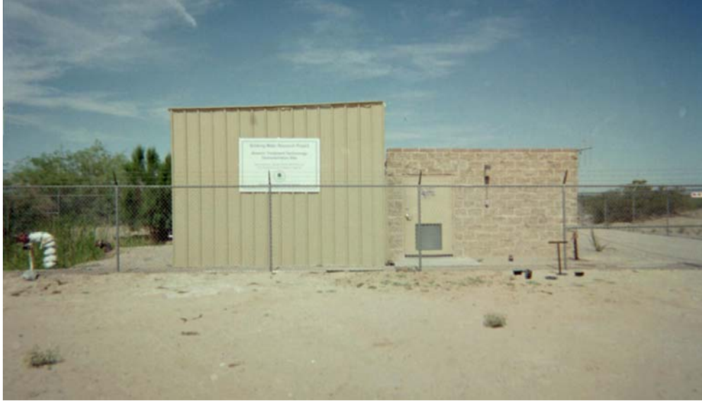
Figure 4-6. Pump House (on the right) and System Enclosure
