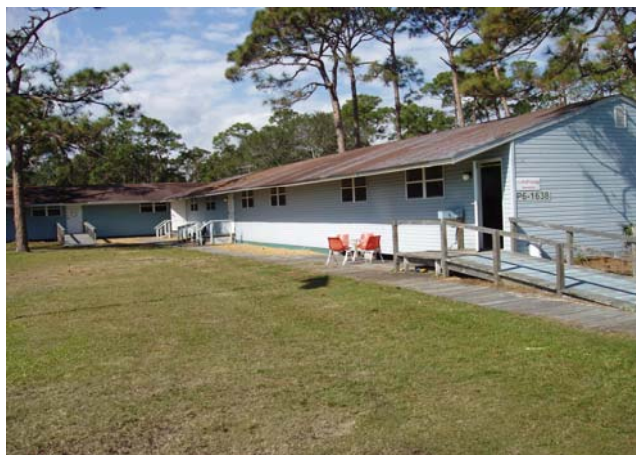
Figure 3-2. KARS Park recreation building.
