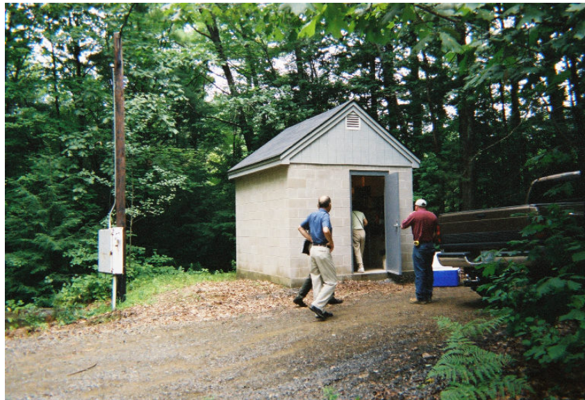
Figure 4-1. Preexisting Porter Well House – Prior to Building Construction and Treatment System Installation
