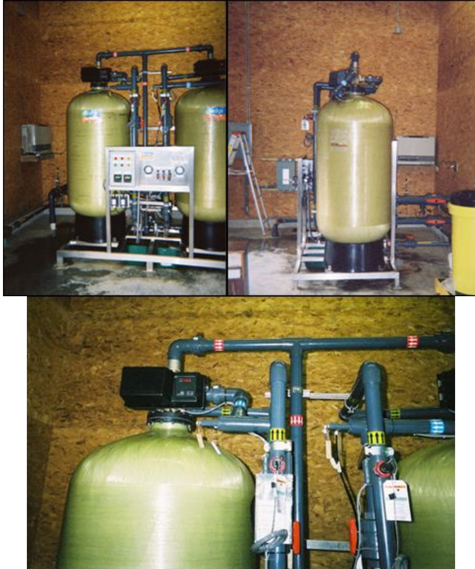
Figure 4-6. APU-100 Treatment System Front and Side View (top) with a Close-up View of Fleck Controller Valve (bottom)
