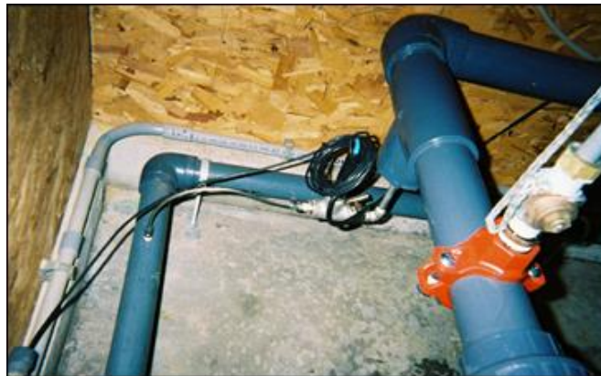
Figure 4-5. Carbon Dioxide Gas Flow Control System for pH Adjustment (From Left to Right: Liquid CO 2 Supply Assembly; pH Control Panel; Sanitary Cross Containing CO 2 Membrane Module; Vault with CO 2 Injection Loop; Port for pH Probe)
