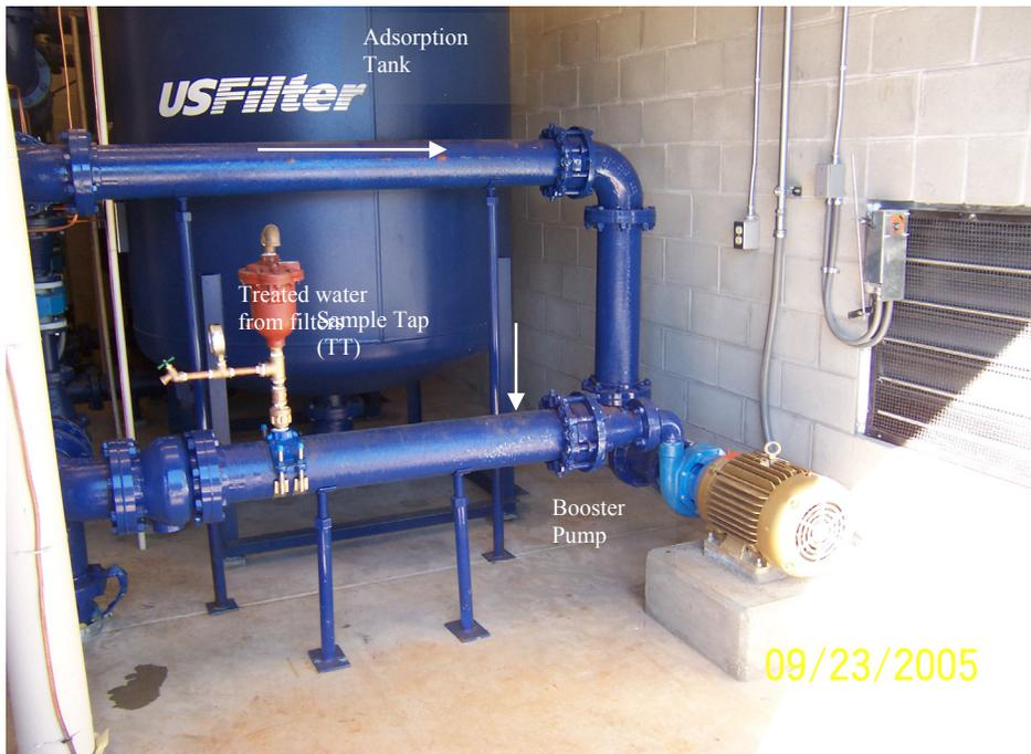
Figure 4-5. A New Booster Pump Station
