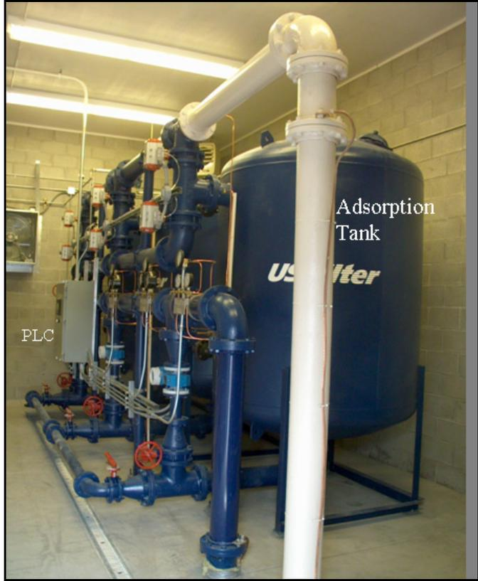
Figure 4-4. Siemens GFH Arsenic/Antimony Removal System
