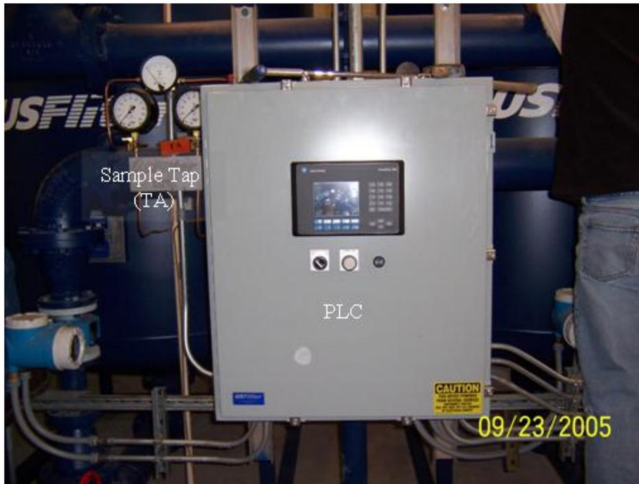
**Figure 4-7. Programmable Logic Controller**
