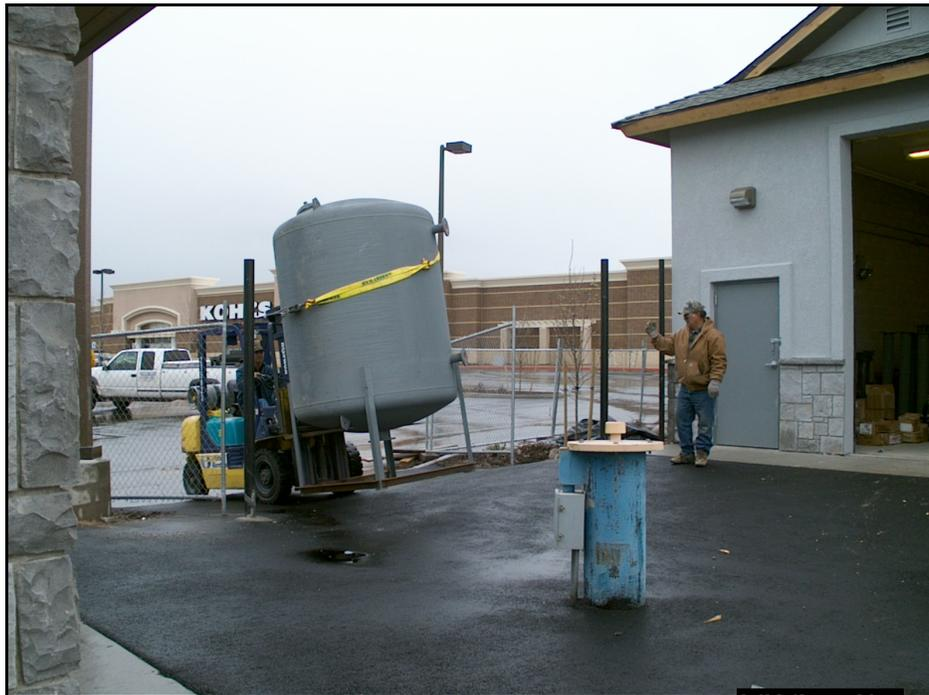
**Figure 4-10. Delivery of One Adsorption Vessel**
