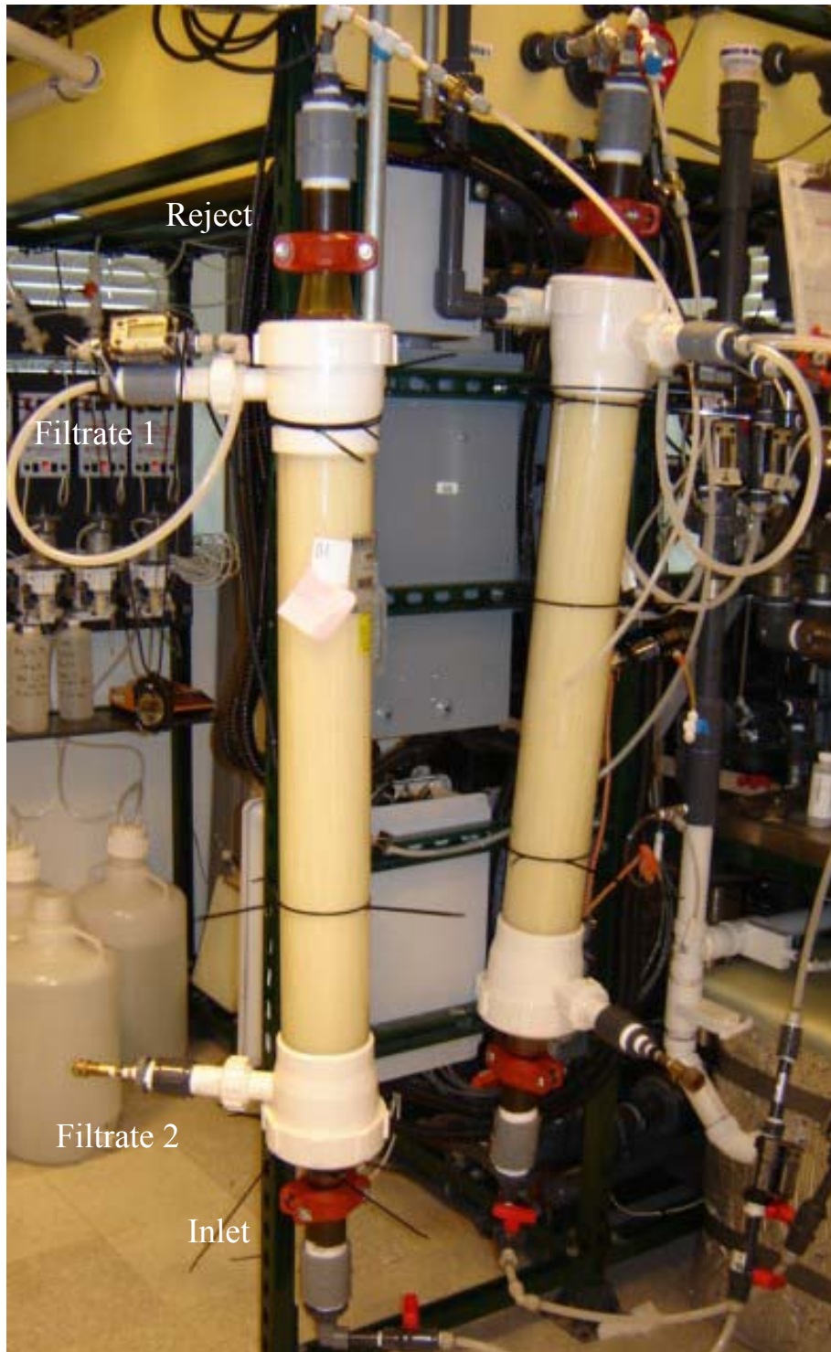
Figure 3-1. UF cartridges plumbed to injection rig test station, showing plumbing connections.
