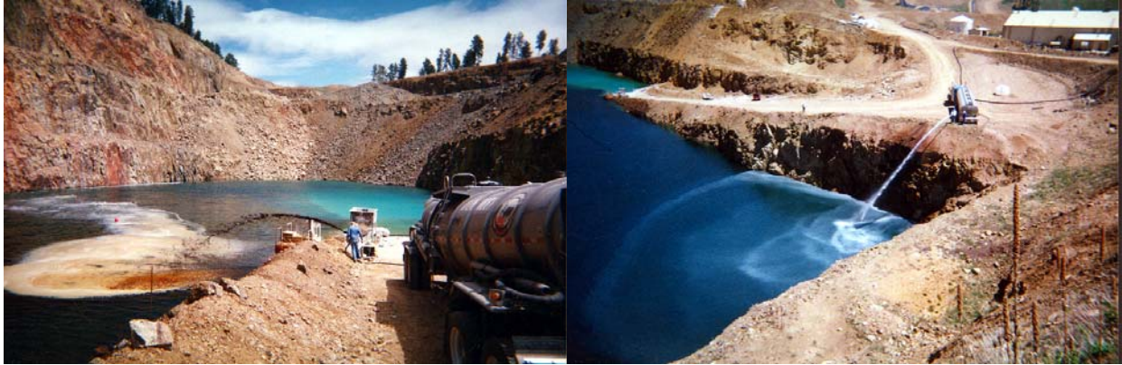
Figure 3-4. Adding molasses (left) and methanol (right) to the pit.
