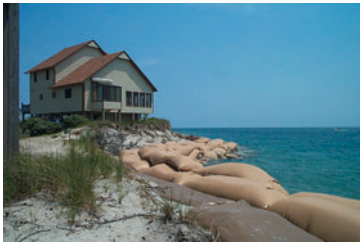
Figure 3.3 On a nesting beach in North Carolina, homeowners placed sandbags to halt erosion, rendering previous turtle nesting sites inaccessible to sea turtles. Photo courtesy of Matthew Godfrey, North Carolina Wildlife Resources Commission.
