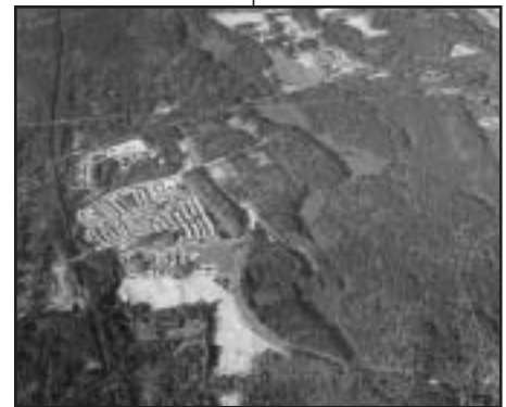
October 2002. Aerial Photo of Redmond Ridge where landscaped areas will be amended to a depth of 12 inches to improve retention of stormwater.
