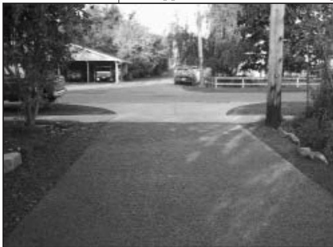
Pervious concrete alley, Bellingham.
