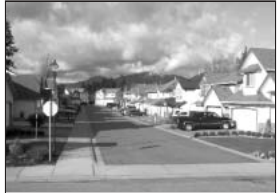
The Peach Road subdivision in Chilliwack, B.C. features small lots, a narrow road and no storm drains in the street.
