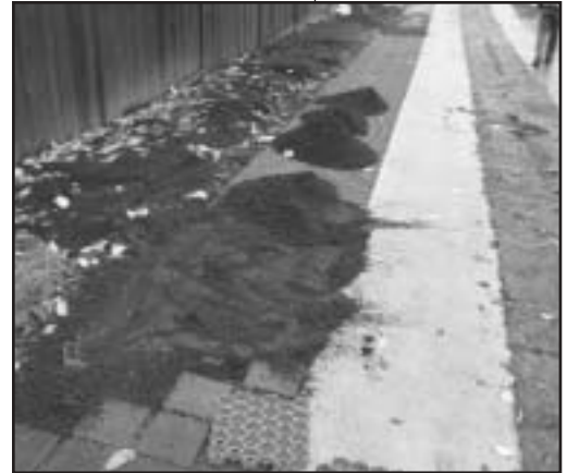
Preparing structural grass.
