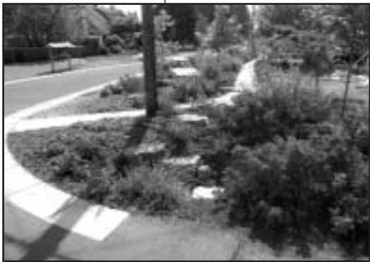
Seattle SEA Streets Project. Graded swales with amended soils reduced stormwater volume by 97 percent for two consecutive years.
