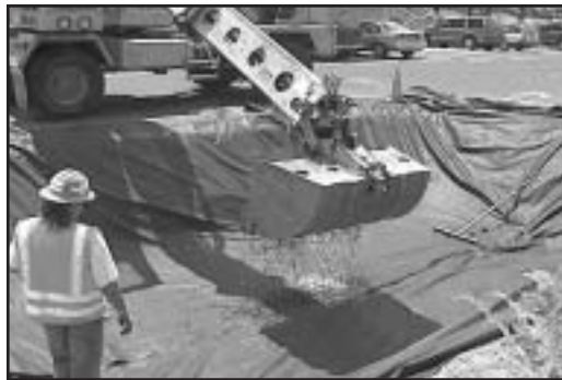
Installing first layer.
