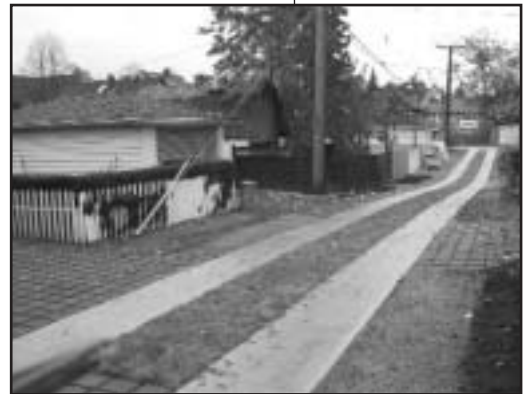
Vancouver Country Lane completed.
