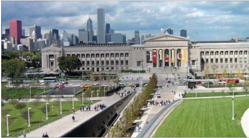
Figure 3-5: Green roof over Soldier Field parking garage, Chicago, IL
