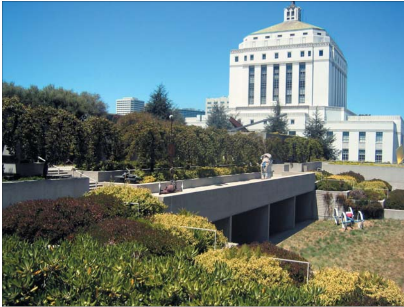
Figures 6-3: A local example of intensive green roofs include the roof-top gardens on the Oakland Museum.
