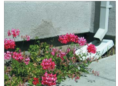
Figure 8-1: Disconnected downspouts drain to planted bio-filtration strips.
