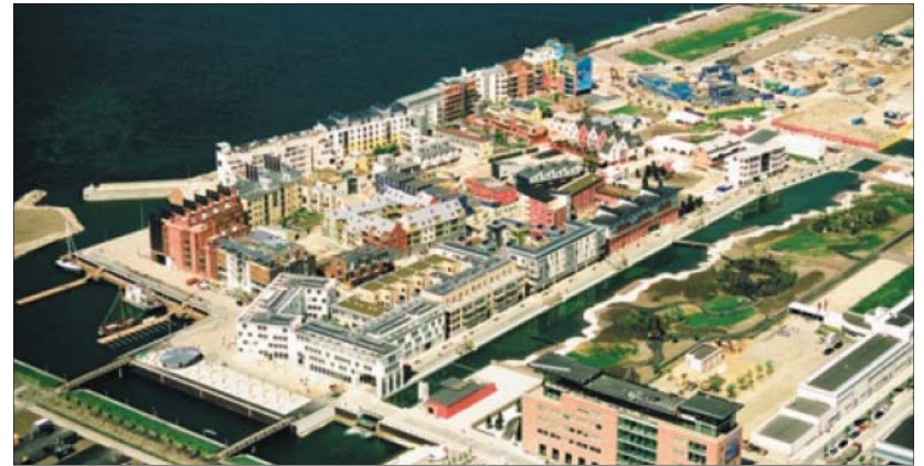
Figure I-1: Aerial photo of green, dense redevelopment on a former industrial site in Malmo, Sweden. This development was created as part of the Bo01 Expo, which showcased sustainable and green design.
