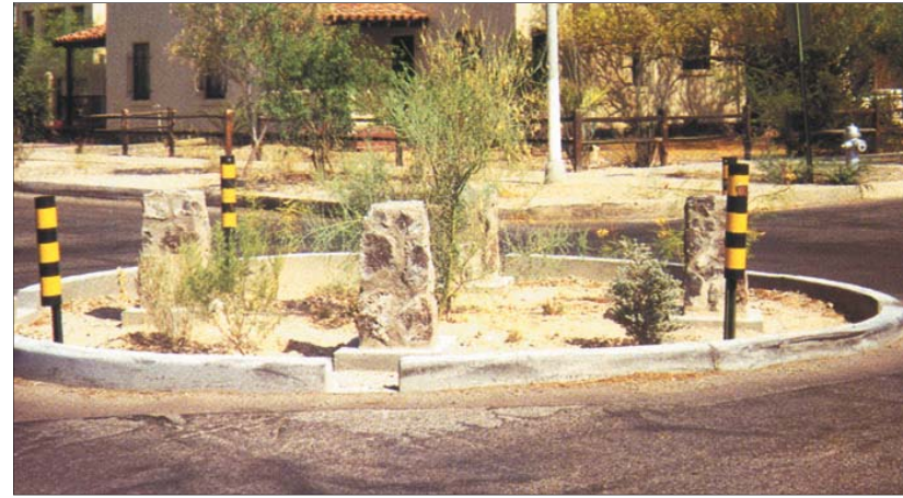
Figure 3-6: Traffic circle and infiltration basin, Arizona
