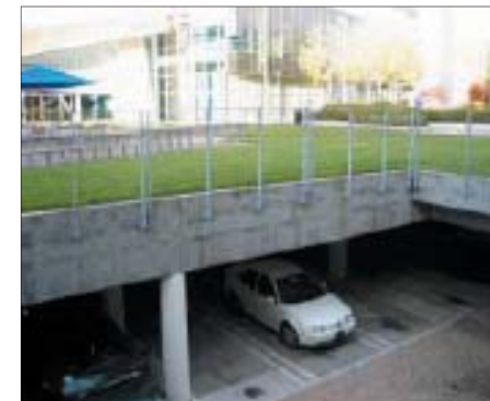
Figure 8-3: Google's green roof deck over parking.
