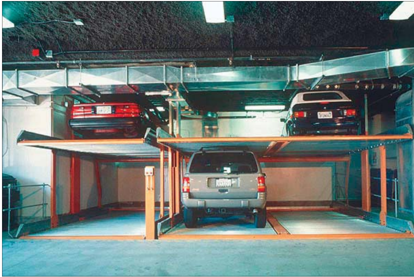
Figure 5-3: Parking lifts maximize the efficiency of parking facilities, resulting in less impervious surface area dedicated to parking.
