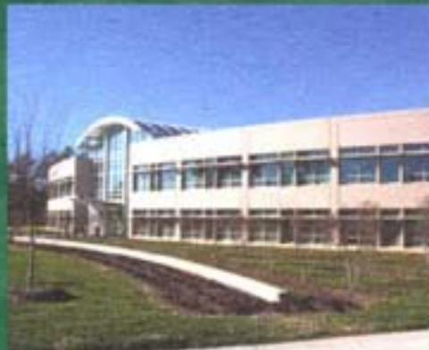
EPA's National Computer Center was designed to achieve a "silver" rating under the U.S. Green Building Council's assessment system - Leadership in Energy and Environmental Design (LEED).
