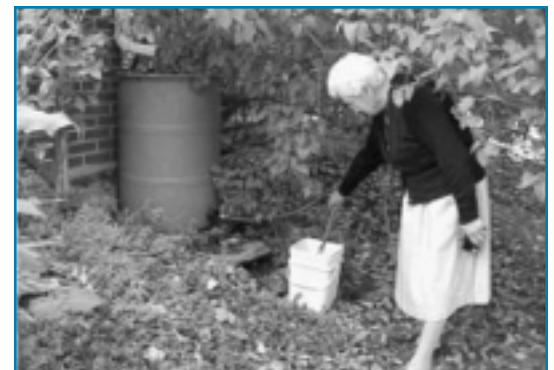
Disconnected downspouts and rainbarrels keep rain out of sewers.
