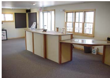
The basis of this cabinetry is a bio-based material created from an abundant agricultural fiber, sunflower hulls bound together with soybean-based resin and sealed with citrus oil.
