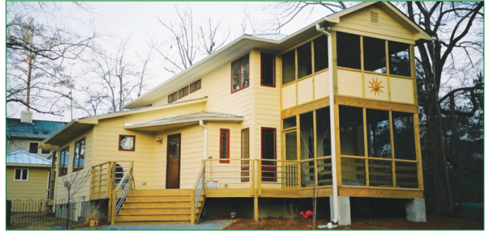
Rick Crume's energy-efficient house in Durham, North Carolina, features south-facing windows to maximize solar heating in winter.
