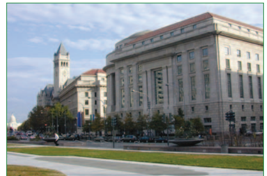
EPA's Federal Triangle complex in Washington, DC, purchased 39 million kWh of green power.
