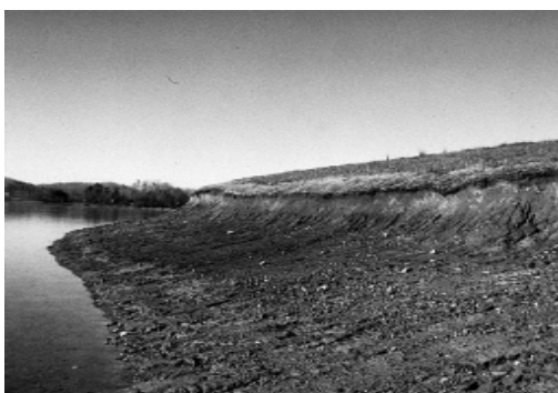
Before—eroding shoreline along TVA's Chatuge Reservoir.
