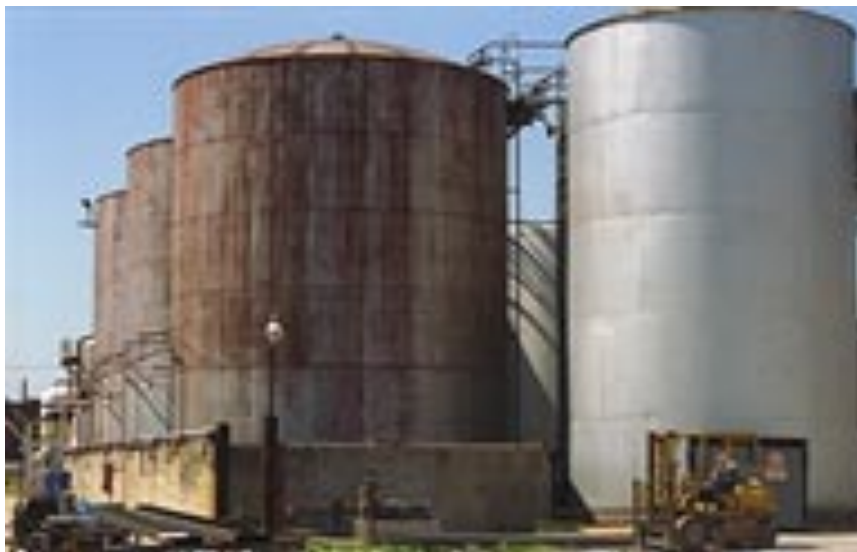
Above is a large vegetable oil storage facility in EPA Region VI.
