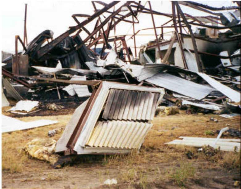
Figure 8. Ventilation Fan with Yellow Residue
