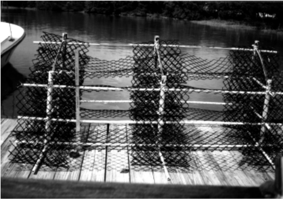
Seawall modules to increase fish habitat
