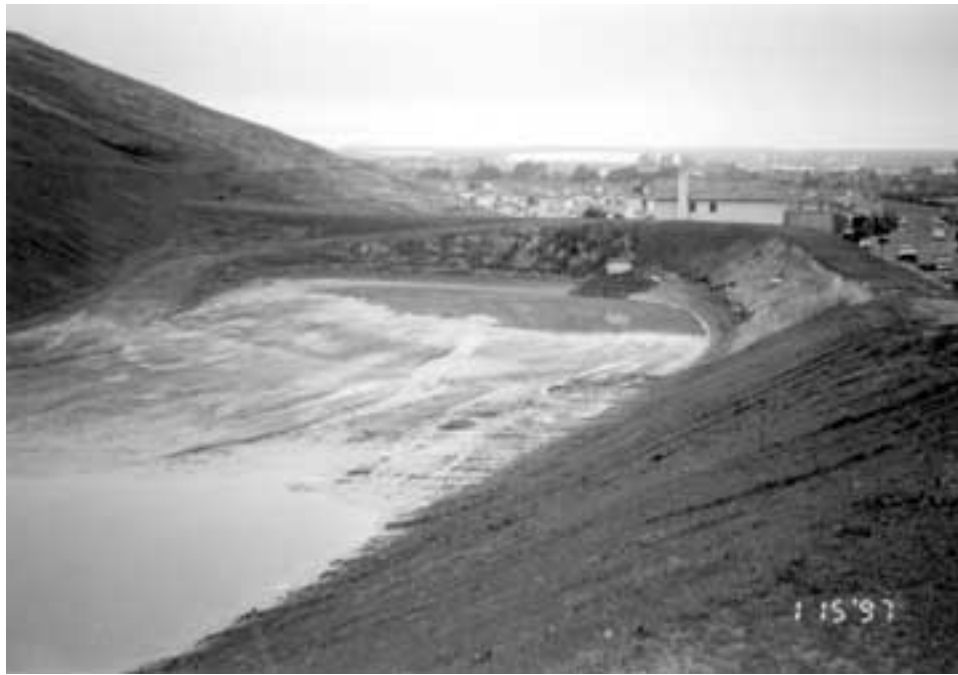
A properly sized sediment basin.
