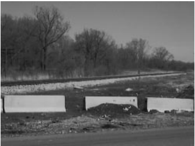
Concrete barriers preventing access along railroad right-of-way
