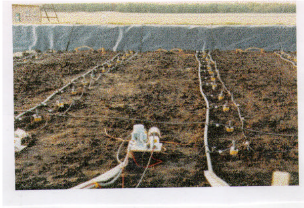
Figure 7 Electrodes in place before power is applied (Source: Geokinetics, International, Inc., Electrokinetic Remediation of Toxic Metals: Statement of Qualifications , June 1997)
