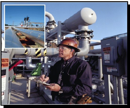
Figure 4: SRS dynamic underground stripping plant for removing solvents from groundwater. (Source: SRS 2001 Annual Performance Report.)
