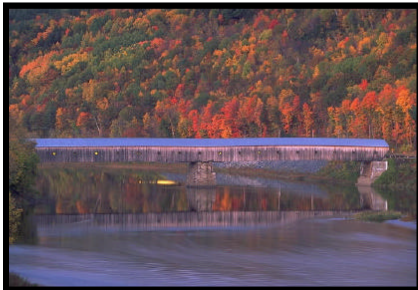
Windsor-Cornish Bridge, Cornish, New Hampshire
