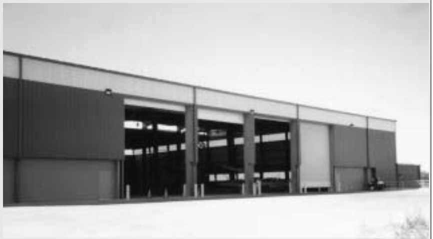
Transfer station structures require tall access doors to accommodate collection vehicles.
