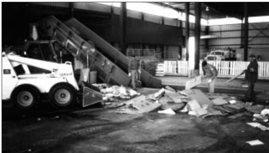
Depositing incoming waste on a tipping floor facilitates waste screening.
