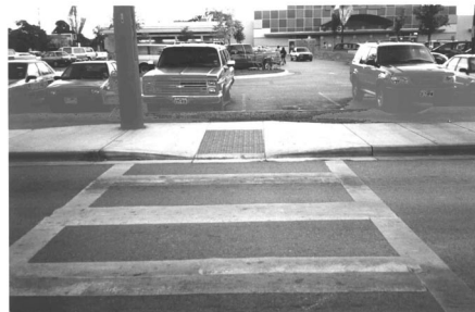
FIG. 5-6. MID-BLOCK CROSSING WITH CURB RAMP, AUSTIN.
