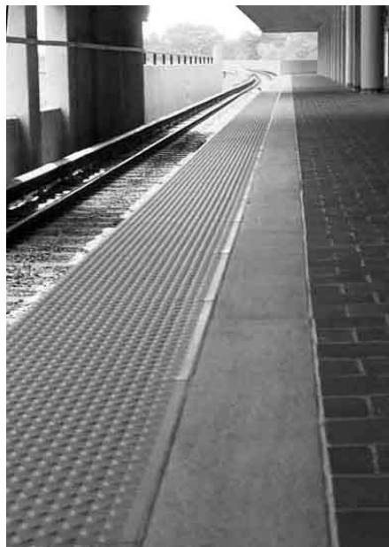
FIG. 2-4. DETECTABLE WARNING SURFACE AT MARTA STATION, ATLANTA, GA.
