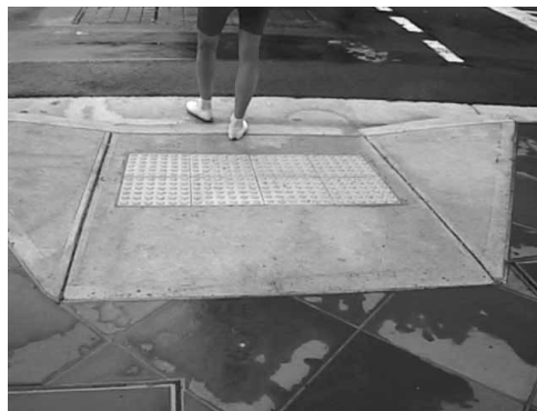
FIG. 4-5. (LEFT) AUSTRALIAN CURB RAMP WITH DETECTABLE WARNING.
