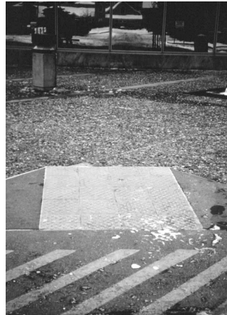
FIG. 5-3. (LEFT) CURB RAMP IN ANCHORAGE, AK.
