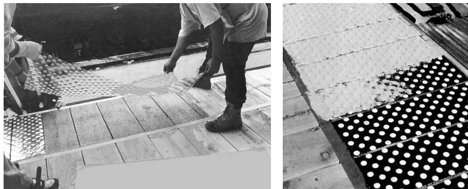
FIG. 7-13. (LEFT) TRUNCATED DOMES ARE ARRAYED ON A CARRIER SHEET (COTE-L).
