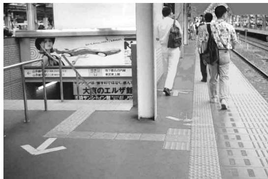
FIG 1-1. JAPANESE TRANSIT PLATFORM SHOWING DETECTABLE WARNING AT THE TOP OF STAIRS AND PARALLEL TO THE PLATFORM EDGE, AND A TACTILE PATH LEADING FROM THE STAIRS TO THE WAITING AREA ALONG THE PLATFORM.
