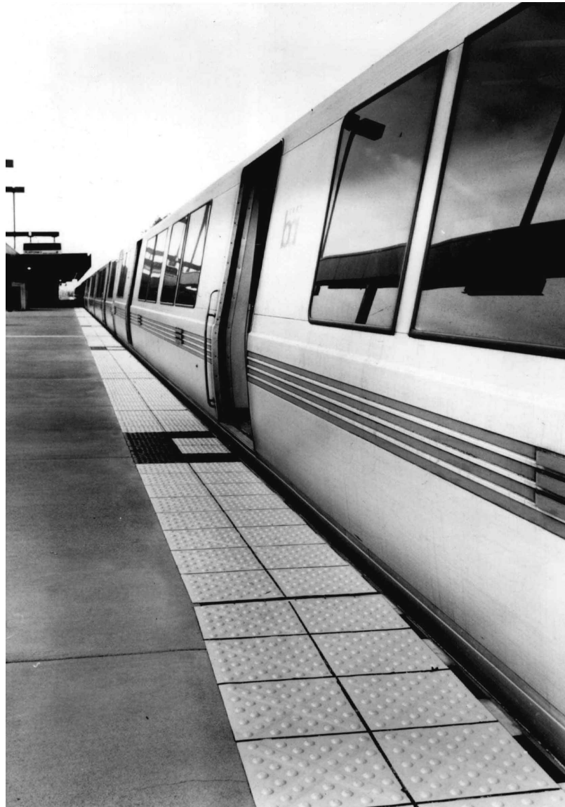
FIG. 5-15. DETECTABLE WARNING SURFACE AT A BART STATION, CALIFORNIA.
