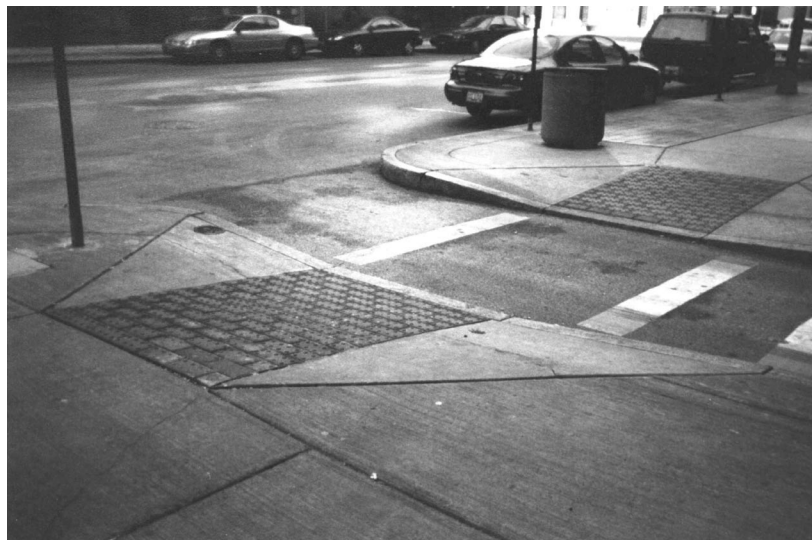
FIG. 1-8. CURB-RAMPS WITH TRUNCATED DOME DETECTABLE WARNINGS ON OPPOSITE SIDES OF AN ALLEY, CLEVELAND, OH.
