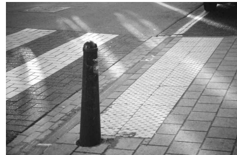
FIG. 4-15. DETECTABLE WARNING PAVERS AT A BLENDED CURB.
