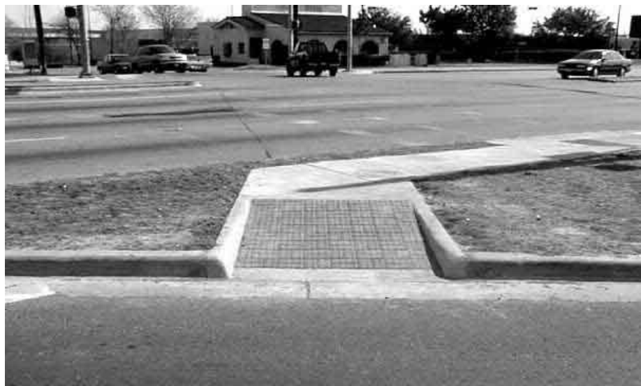
FIG. 6-2. SPLITTER ISLAND WITH DETECTABLE WARNING ON FULL SURFACE OF CURB RAMP, AUSTIN, TX.
