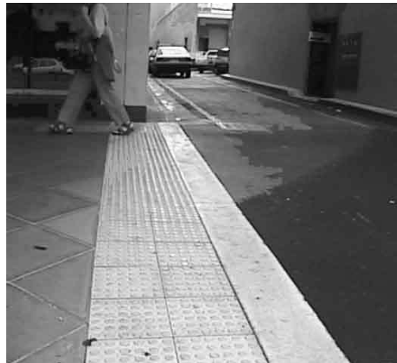
FIG. 4-7. DETECTABLE WARNING SURFACE ACROSS FULL WIDTH OF SIDEWALK AT AN ALLEYWAY (HAZARDOUS VEHICULAR WAY) IN AUSTRALIA.
