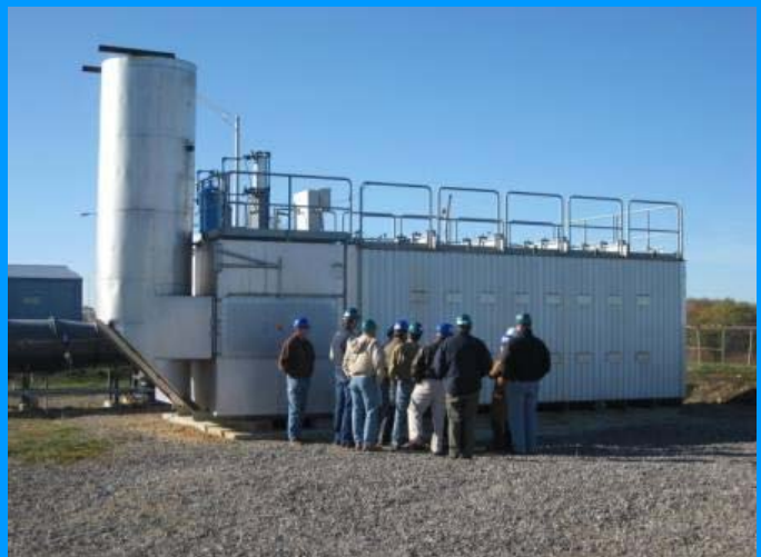
CONSOL Energy hosted a site tour of its technology demonstration project featuring the MEGTEC VOCSIDIZER at an abandoned mine site in West Liberty, WV.
