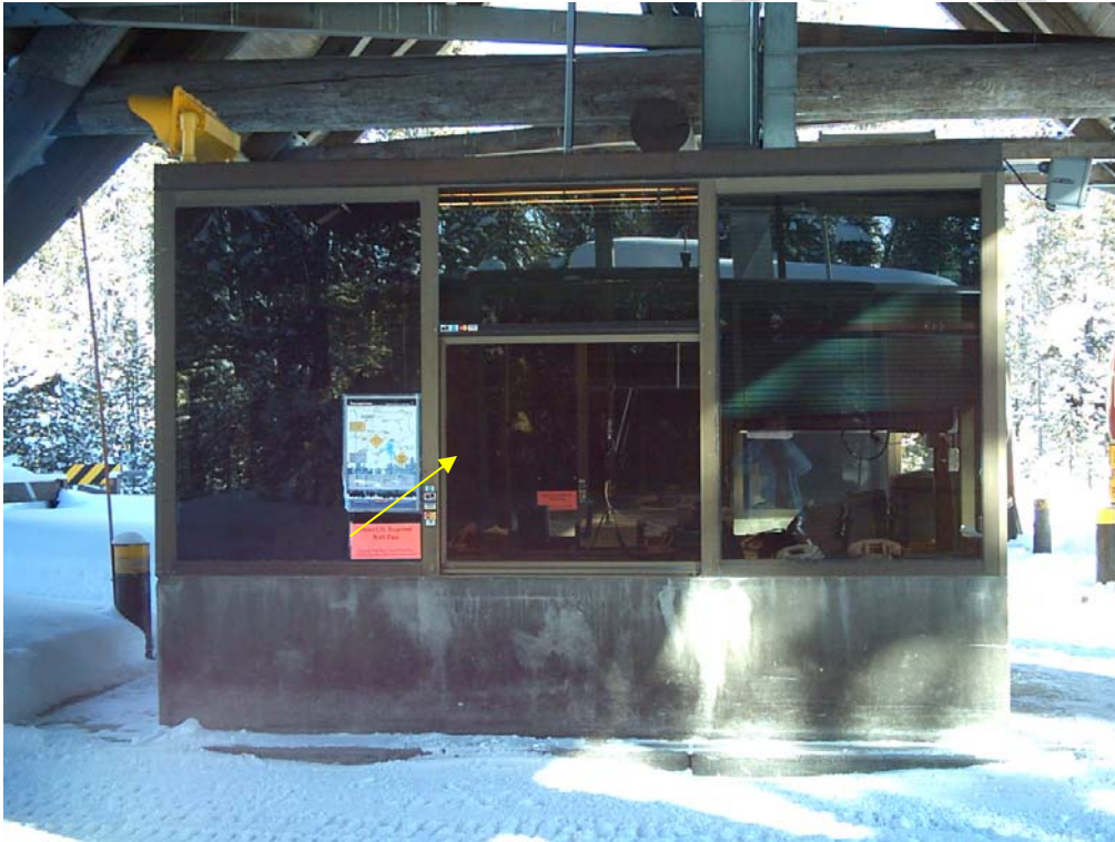
Figure 4. Location of mini-can area samples in kiosk A at the West Entrance
