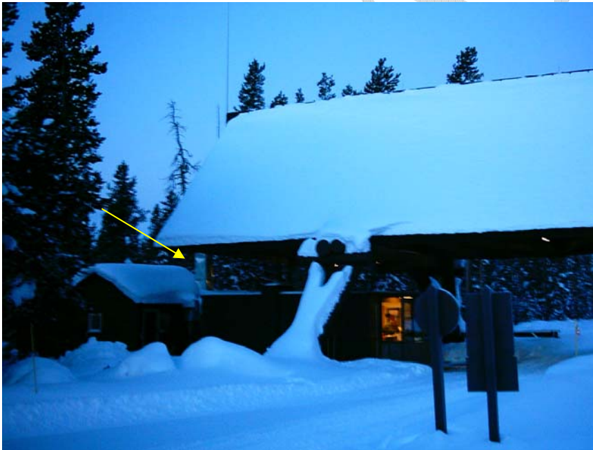
Figure 6. Ventilation duct to West Entrance kiosks
