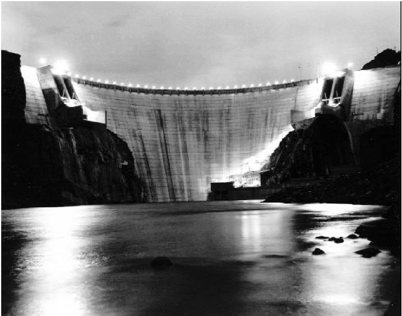
Theodore Roosevelt Dam, Central Arizona Project, was re-dedicated in April, 1996, following completion of Safety of Dams modifications (photo by Reclamation).
