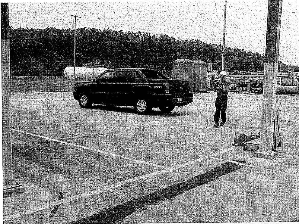
Spill Area Asphalt Cap – truck parked on cap – delineated by yellow lines
