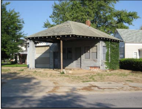
An abandoned gas station along the Lincoln Highway in Jefferson, Iowa.
