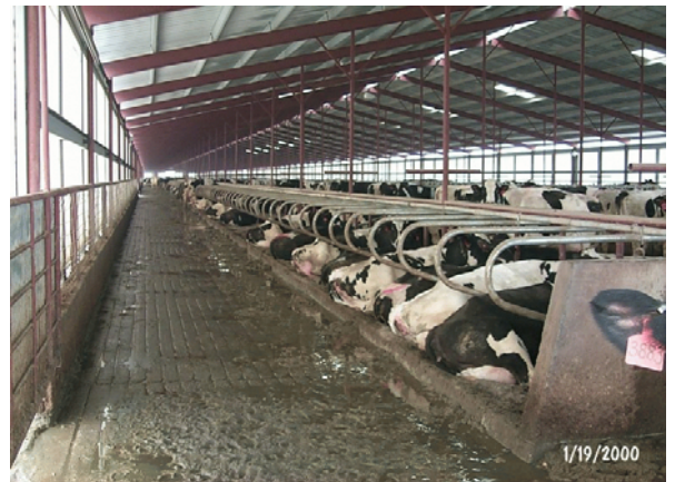
Flush-dairy manure channel
