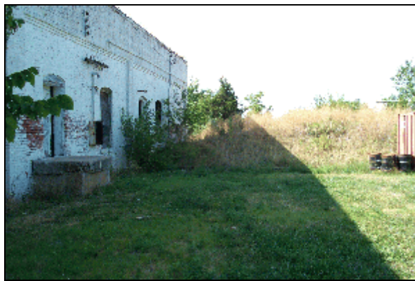
Chemical Commodities, Inc. building and stockpiled soils, 320 S. Blake, Olathe, Kansas.
