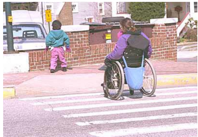
Curb ramps provide basic access at intersections and pedestrian crossings.
