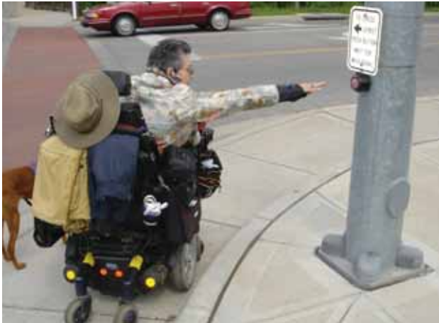
This new parallel curb ramp on a large-radius suburban corner curves down to the street and is otherwise usable, but the pedestrian isn't. Installed on a signal pole, it is out of horizontal reach range for this pedestrian. A better installation can be seen across the street, where a stub pole has been installed in a more usable location.
