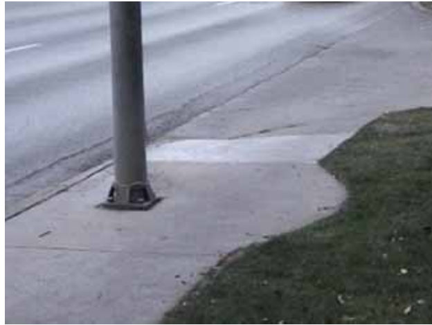
Photograph of a sidewalk widened to go around an obstruction.
