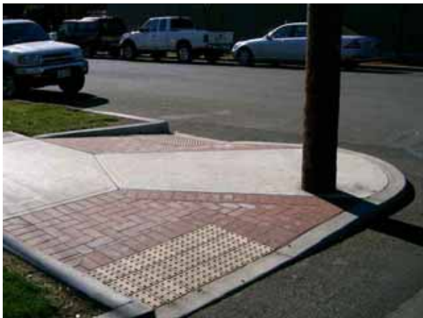
Curb ramp with returned curb adjacent to landscape strip
