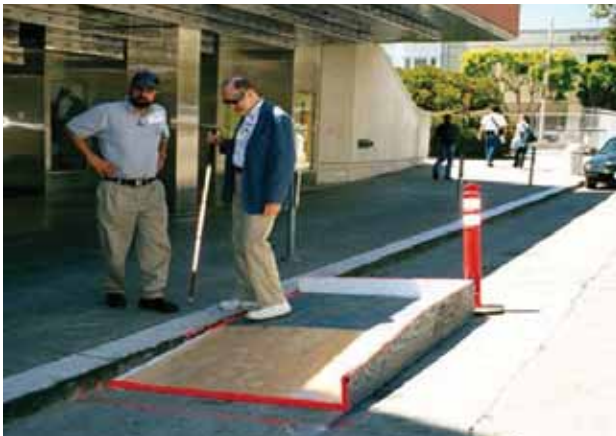
San Francisco uses plywood curb ramps with edge protection for temporary sidewalk detours. Here PROWAAC member Ken Stewart of CCLVI (with white cane) tests a model while Lukas Franck of The Seeing Eye looks on.
