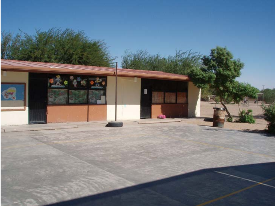
Figure 7. School in La Grullita. Monitor was placed in Director's Office.-
